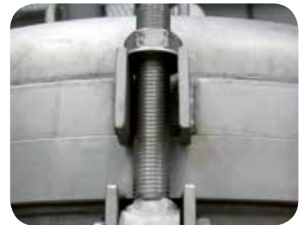
Details of the hinged nuts.
